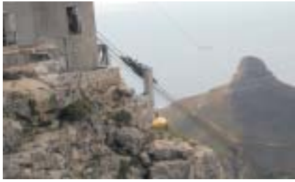
Upper Cable Station
